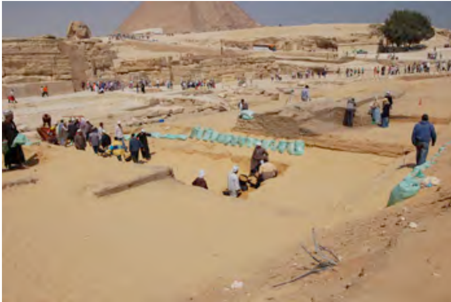
View of excavation trench in front of Khafre's valley temple (Photo: SCA)
